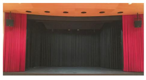
• Above L-Acoustics X12's are used as the main PA and the 5XTs are mounted on the rear wall for cinema applications. all of which are powered by an LA4X amplified controller. A further four X12's are used for monitoring, one of which is also used as a centre speaker for cinema applications along with four 5XTs positioned on the rear wall.
